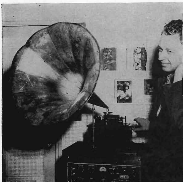
The ancestor of modern horn-type enclosures is this 19th century "Morning Glory."
